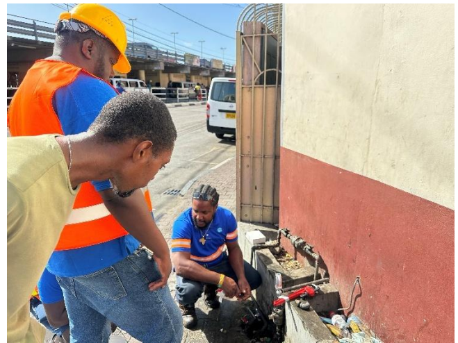
Auditors at the St. George's Medical Center inspecting pipe fixtures
