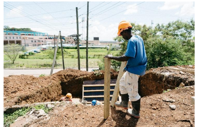
Hospital Laundry Cistern Under Construction
