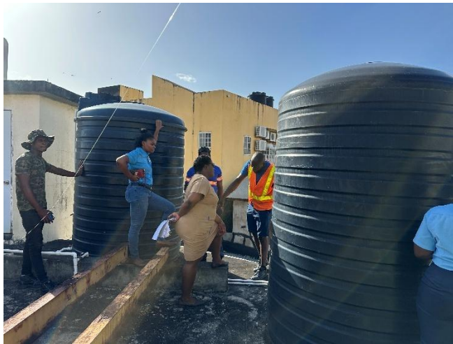
Water Storage tank inspection during audit
