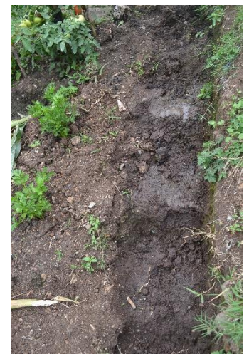
Drain on the slope with steps to slow down the flow of water, HM Prison's Farm, St George
