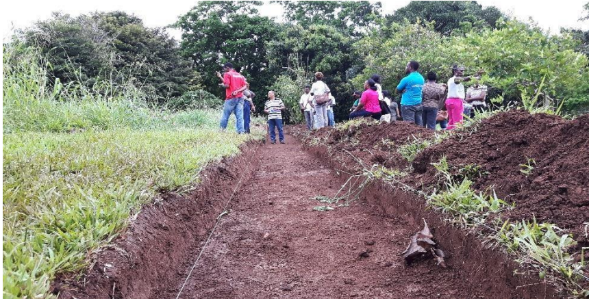
Building a drain at the Mirabeau Propagation Station, St Andrew
