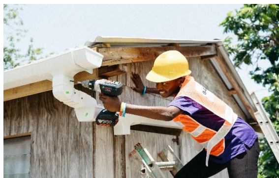
GWAP Member Ronda Stafford installing spouting on recipient home
