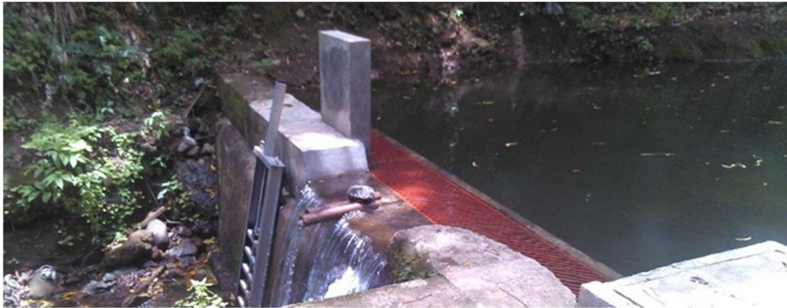
Figure 12. Improved water intake at Mont Reuil water intake (“Tyrolean weir” type grille with slatted horizontal water intake pipe inside the weir)
