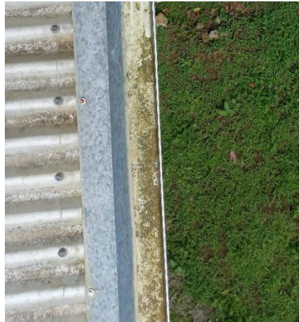
Figure 5.3 - Photo showing drip edge installed to improve collection of water into guttering
