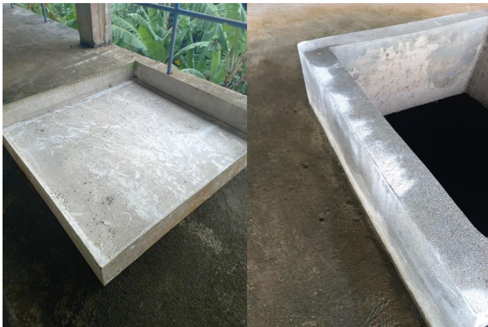
Figure 6.2 - Photos showing powder substance under manhole covers and manhole walls
