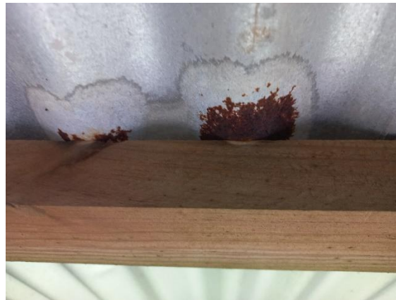
Figure 4.3 - Photo showing corrosion to the underside of roof sheeting where it sits on purlins
