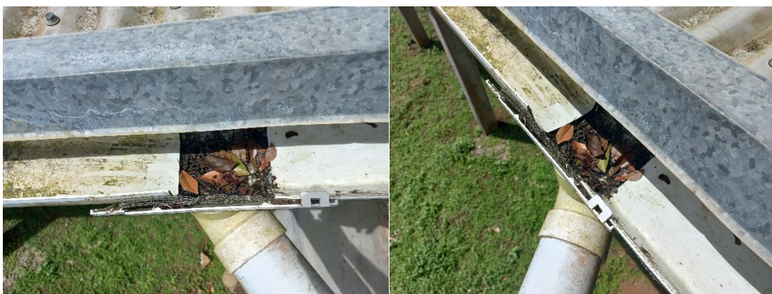
Figure 4.1 - photos showing leaves in guttering at Blaize.
