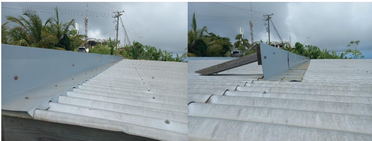
Figure 5.2 - Photos showing "L" shaped rain stops installed to prevent rainwater flying away
