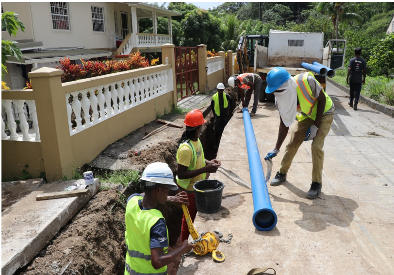
Workmen installing new pipelines in the parish of St. Mark
