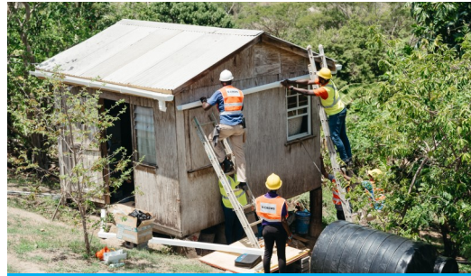
Members of GIZ & GAWP installing spouting on recipient home
