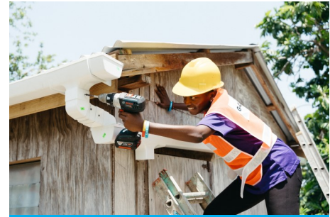
A GAWP Member installing spouting on a recipient home
