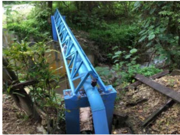
Figure 15: Fortified pipeline river crossing; source: USAID, 2017 xviii
