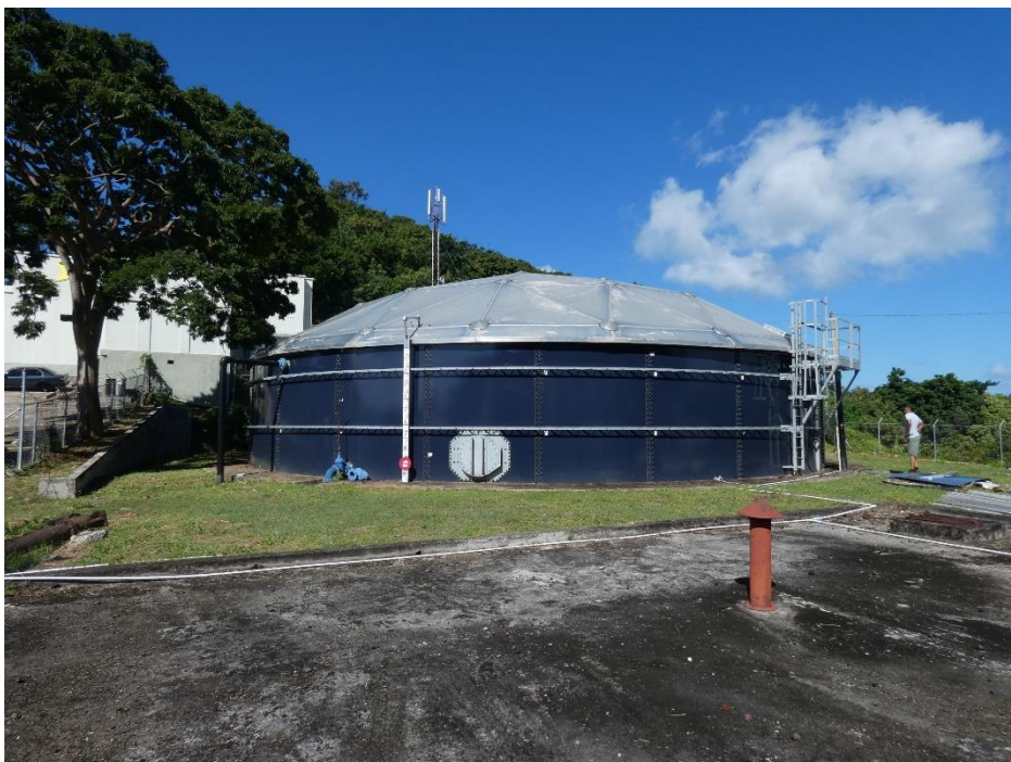
Figure 7: Water tank in Grenada, 2021, © GIZ Grenada / Marion Geiss
