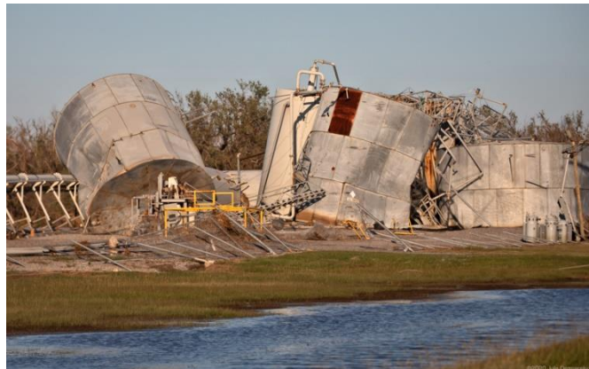
Figure 10: Destroyed tanks after high wind speeds due to a hurricane, © DeSMOG / Julie Dermansky
