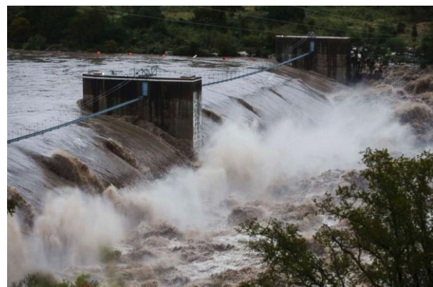
Figure 20: Dam during a flood event; source: ABC News; https://abcnews.go.com/
